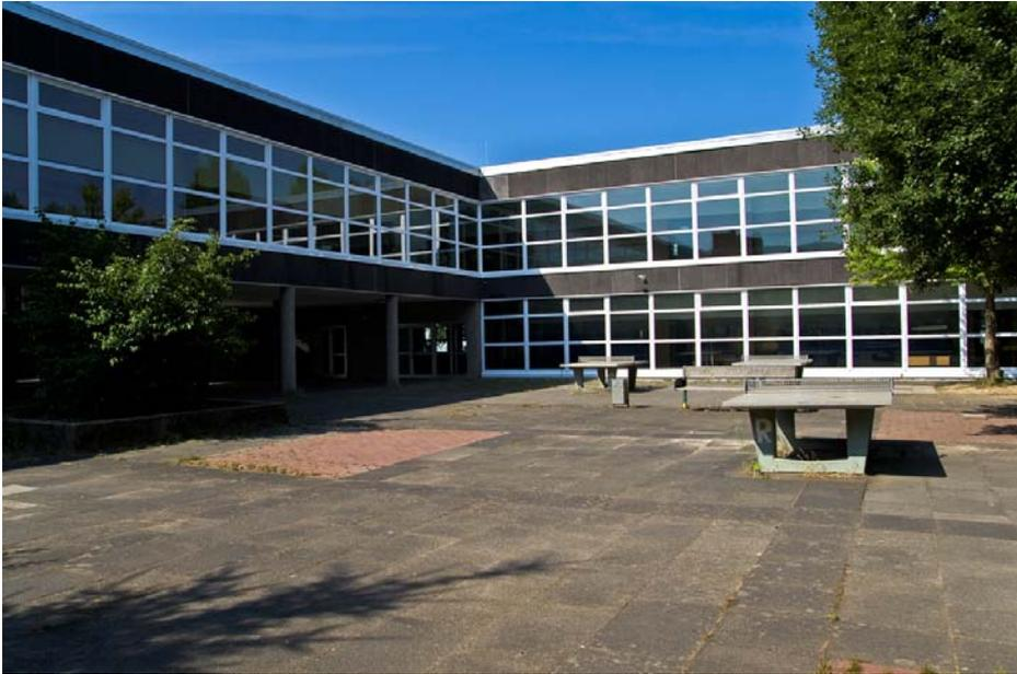
Tomburg intermediate secondary school, interior view: The circumferential façade in the patio of Tomburg intermediate secondary school was particularly challenging due to the lintel section without load-bearing capacities. "InnoNova 70" system offered a suitable solution.
