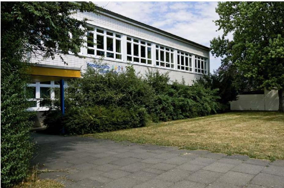
Primary school Sürster Weg: The existing steel windows could not be removed so that the remaining steel frames had to be superstructured. Thus, the slim aspect of the Trocal profile system was preserved just as its excellent thermal insulation properties.
